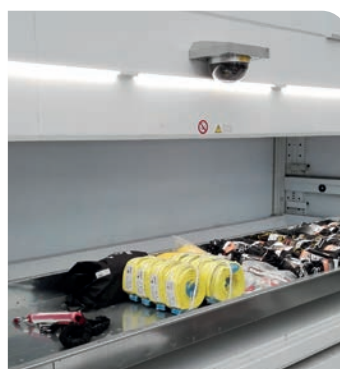
External bay lighting
